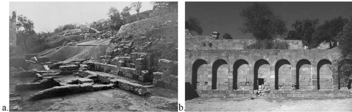
Figure 3.14 View of the Main Hall of the library: a) before its restoration (Laurenzi 1938, pl. 18); b) after the restoration of the niches (Hoepfner 2002, fig. 72).
