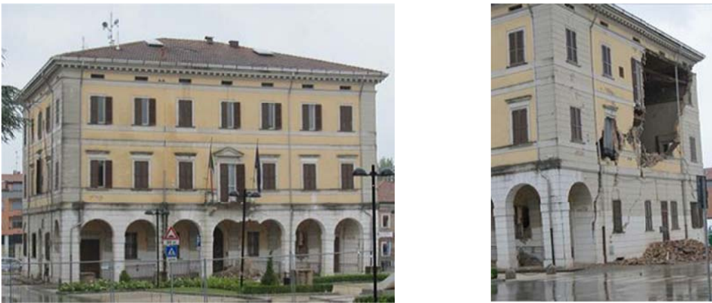
Figure 1.2 Building damage after the Emilia earthquake (Decanin et al. 2012)
