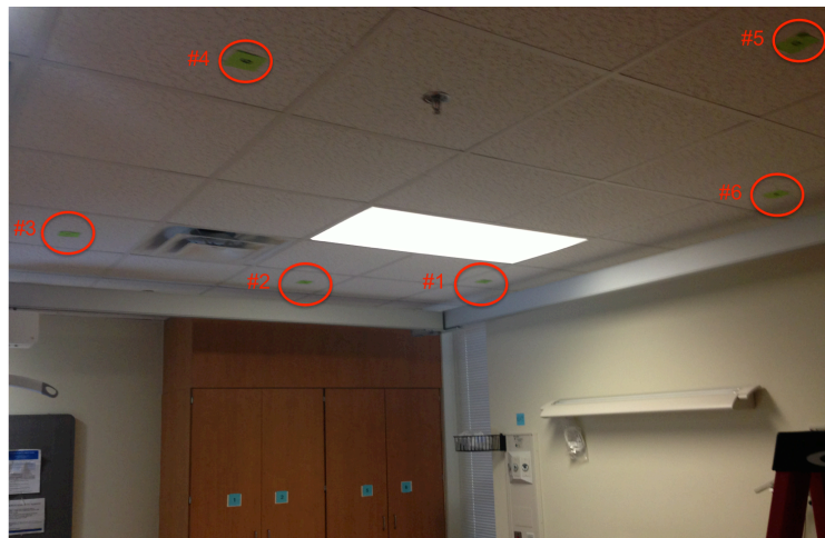
(c) HVAC-tiles labeled from 1 to 6 on the roof
