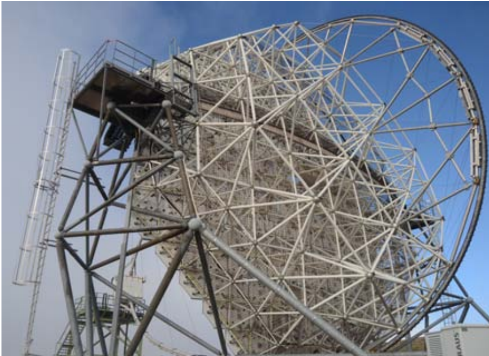
Figure 3.5: Back of the structure of MAGIC-I telescope. White carbon fibre tubes compose the main frame. The counterweights are placed in the curved back part of the arch.
