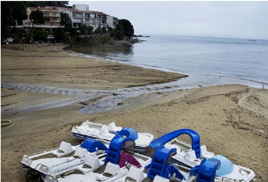
Figure 26. Signs of overwashed beach due to storm event in Roses. Source: Author, 2012
