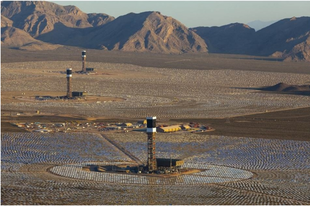
Figure 1.10: Photo of Ivanpah solar power facility using central collector system ([11]).
