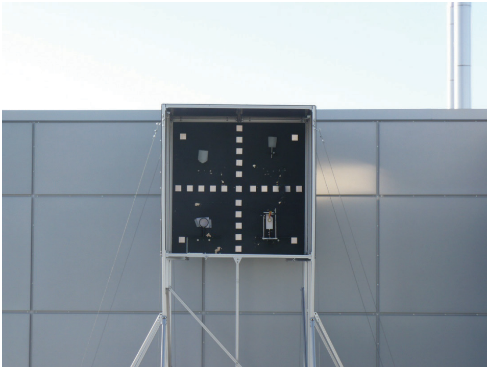
Figure 47 – Close Up of Target Box Structure.
