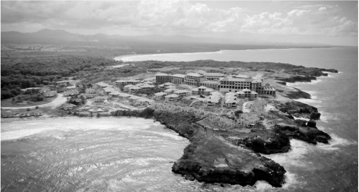
Image 6-4: Roco-Ki Deserted Mid-Construction. Source: Own Photograph. Taken May 1, 2011.
