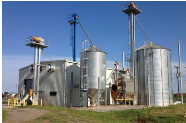
Figure 8. Crop Processing Facility.
