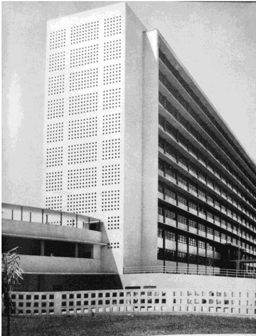
FIGURE 9.36 Lathrop Douglass, Architect, Edificio Creole, Caracas, 1954. East facade, protected with camdogés , and north, with visors. Source: Architectural Record (June 1955), 149.
