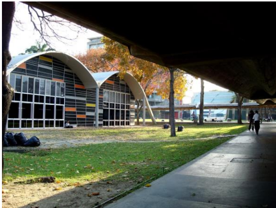
FIGURE 7.19 C. R. Villanueva, University City. The Engineering Library, with mural by Alejandro Otero (view from one of the passages of the covered walk system). Notice in the background the Main Library (tall tower block). Source: photo by Jorge Villota P., 2009.
