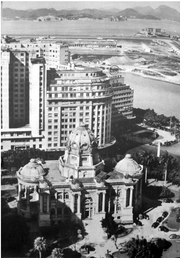
FIGURE 2.16 Robert R. Prentice, Headquarters of the Brazil Division of Standard Oil (with an Esso sign atop), 1932, located in the photo between the Monroe Palace (foreground) and the Santos Dumont Airport (background). The U.S. Embassy Building was located behind the round-cornered edifice. Source: The Lamp (Sept. 1954), inner cover.
