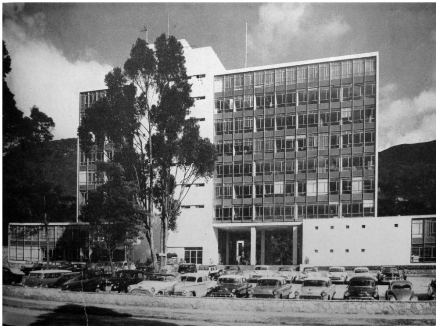
FIGURE 9.11 Lathrop Douglass, Architect, Edificio Esso for Colombiana, S.A., Bogotá, 1956. Rear façade and parking area. Photograph by Paul Beer. Source: Architectural Record (Mar. 1958), 167.
