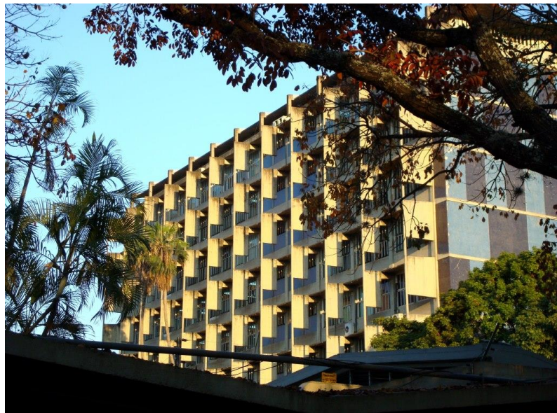
FIGURE 7.33 C. R. Villanueva, University City, School of Architecture Building, 1954-1957. Façade with brise-soleils ; mural by Alejandro Otero. Source: photo by Jorge Villota P., 2009.
