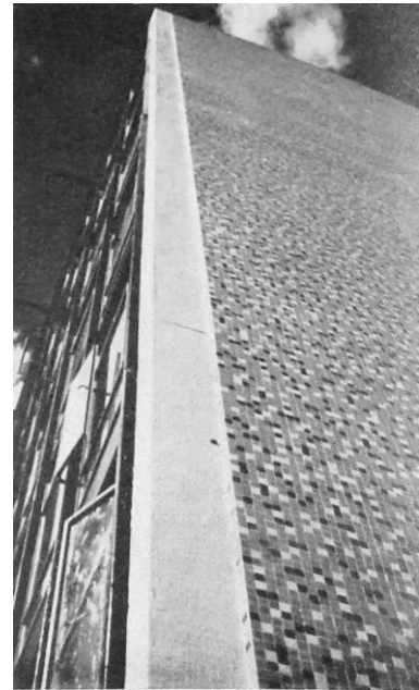
FIGURE 9.14 Lathrop Douglass, Edificio Esso for Colombiana, S.A., Bogotá. Colored ceramic tiles on lateral facade. Source: Architectural Record (Mar. 1958), 170.
