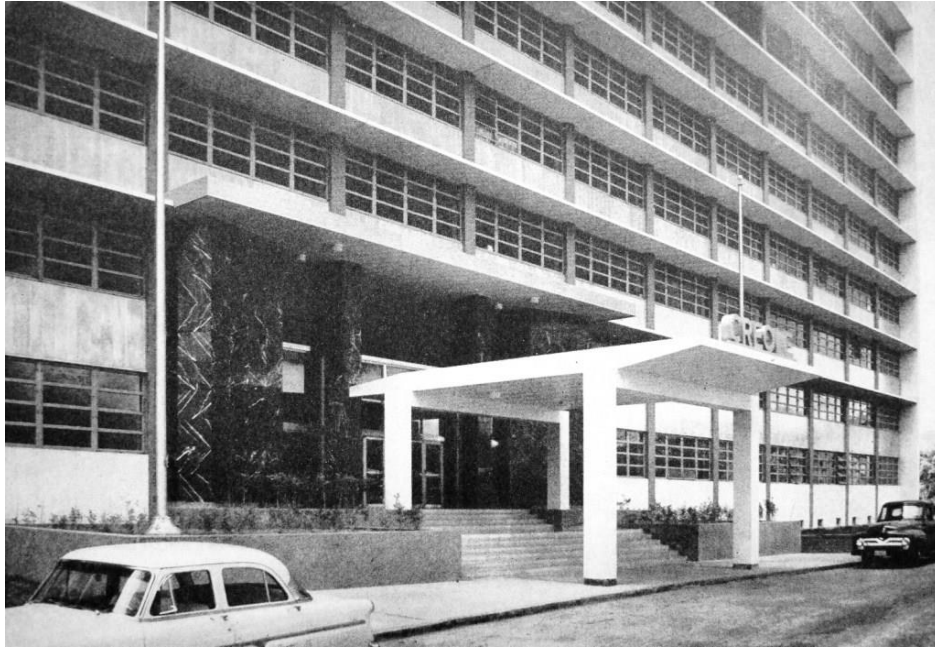
FIGURE 9.44 Lathrop Douglass, Edificio Creole, Caracas, 1954. Main entrance, at the north façade. Source: Architectural Record (June 1955), 152.
