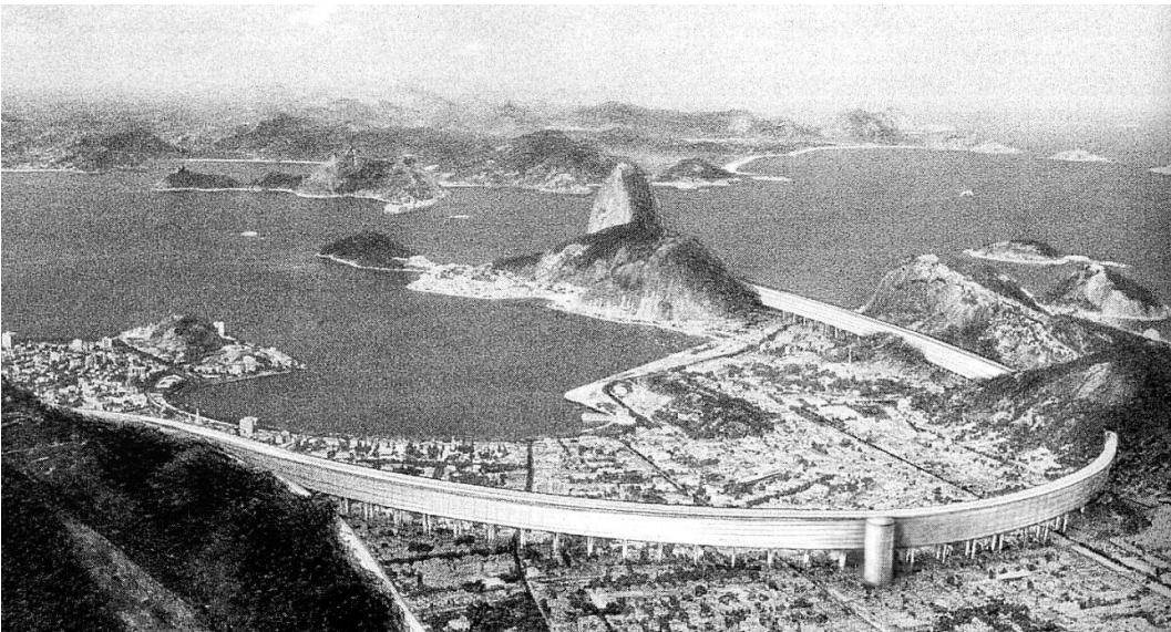
FIGURE 11.36 Le Corbusier, extension for Rio de Janeiro, 1930 (photomontage). A highway on top of curving housing building. Source: Tsiomis (1999).
