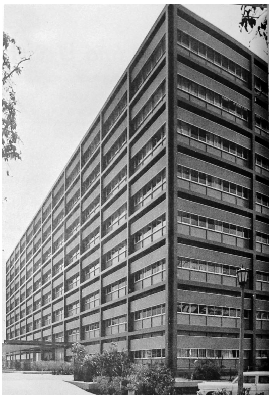
FIGURE 4.20 Don Hatch, Mobil-Oil Office Building, Caracas, Venezuela, completed 1959. Source: Venezuela Up-to-date (Nov. 1959), 14.
