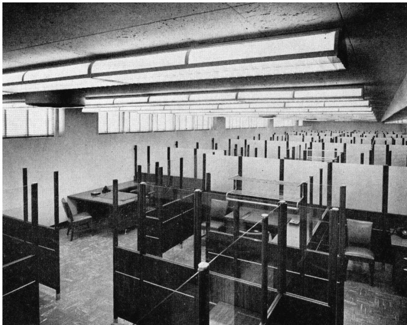
FIGURE 9.26 Lathrop Douglass, Standard Oil Company Refinery Office (Bayway Office Building), Elizabeth-Linden, New Jersey, 1953. Partitions between private and semiprivate offices, and between departments. Windows had sills 6 ft. 6 in. above floor level. Source: Architectural Record (Apr. 1954), 209.
