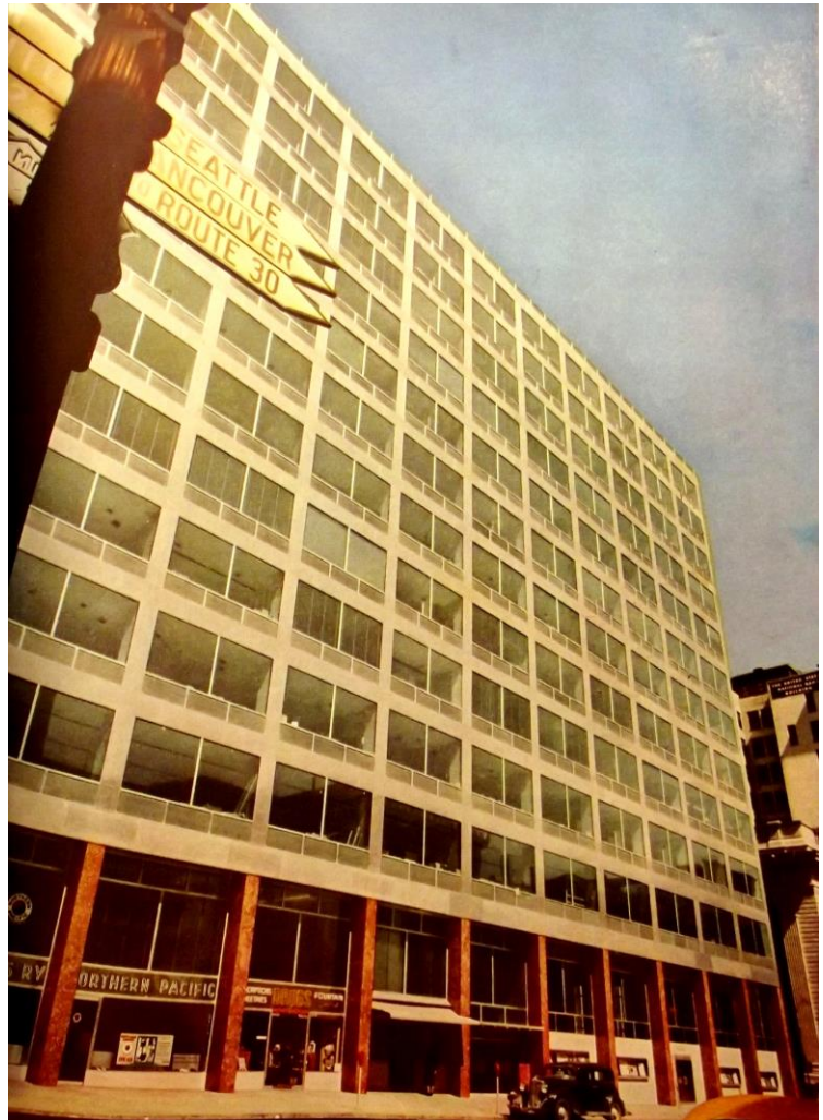
FIGURE 2.3 Pietro Belluschi, architect, Equitable Saving & Loan Building, Portland, Oregon, 1948. Its huge areas of sea-green glass not only reduced solar heat, but also to cut down sky glare to a point where blinds or shades were not needed for comfort. Source: Architectural Forum (Sept. 1948), 101.
