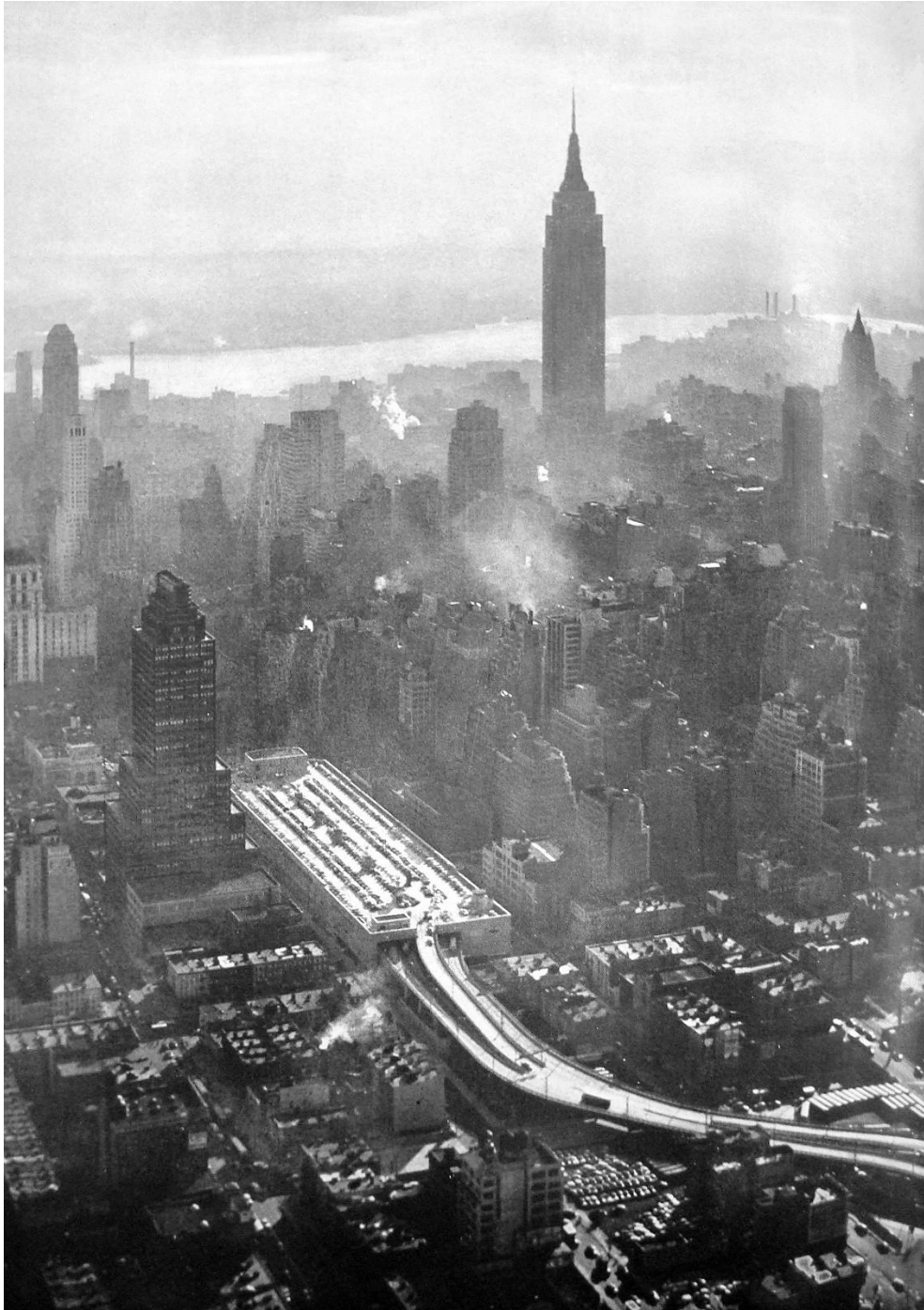
FIGURE 1.21 Manhattan's Bus Terminal, New York City, 1949-50. The roof of the building provided parking space for cars from the Lincoln Tunnel. Source: The Lamp (March 1954), 20.
