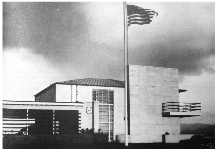
FIGURE 7.6 New Residence of the U.S. Ambassador in La Florida neighborhood, Caracas, where Mr. and Mrs. Fletcher Warren received the Good Will Mission from Fort Worth, Texas, in June 1952. Mr. Warren had moved to this building that very same month. Source: Venezuela Up-to-date (July-Aug. 1952), 21.
