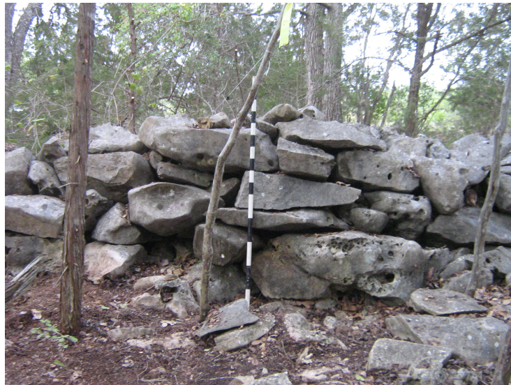
Figure 5.3: Picture of stacked tabular limestone slabs on one section of the rock walls (Photo by Doug Boyd, 2009).
