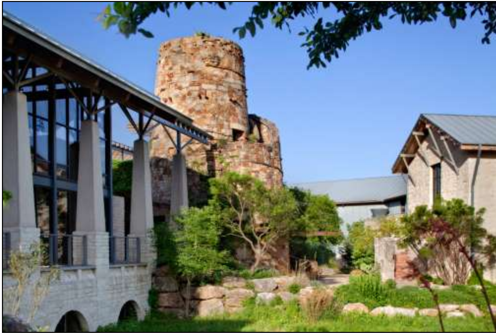
Photograph 113: The Lady Bird Johnston Wildflower Center provides an exemplary example of how buildings can be designed to reflect the ecological and cultural history of their regions.
