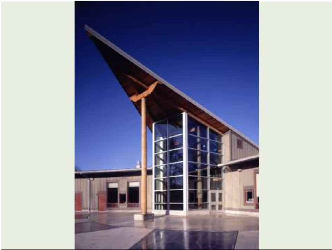
Photograph 98: Designed to portray a thunderbird watching over territorial lands, the design of the Wa He Lut Indian School entryway incorporates traditional heritage and sends a message of community values.
