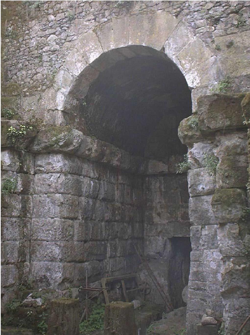
Figure 4.33 The Albano Emissary, vault leading into tunnel (Photo B. Robinson, with permission)
