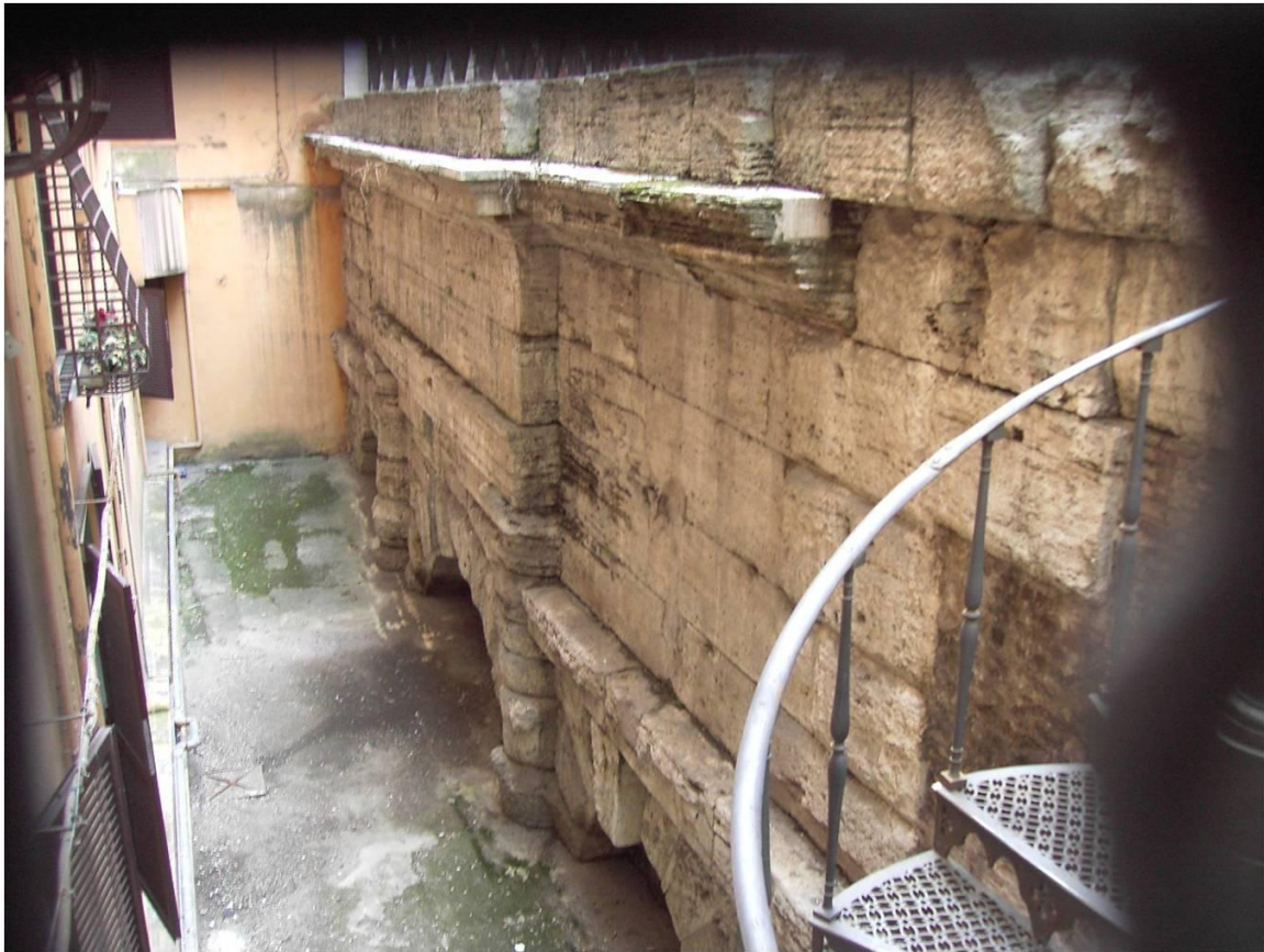
Figure 3.20 Arcus Claudii in Via del Nazareno. Because it is only partially excavated and tightly enclosed on all sides, the monument is very difficult to photograph. (Photo Joelle L. Lardi 2009)
