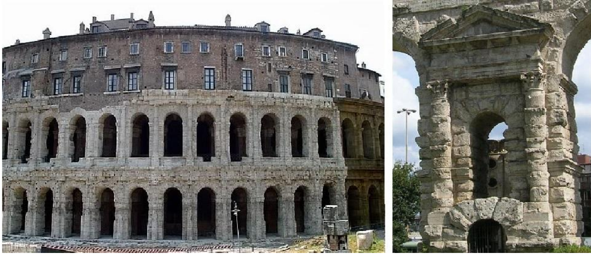
Figure 3.29 Comparison between the rusticated styles of the Theatre of Marcellus (completed 13 BCE) and the Porta Maggiore (52 CE) (Photos Joelle L. Lardi 2009)
