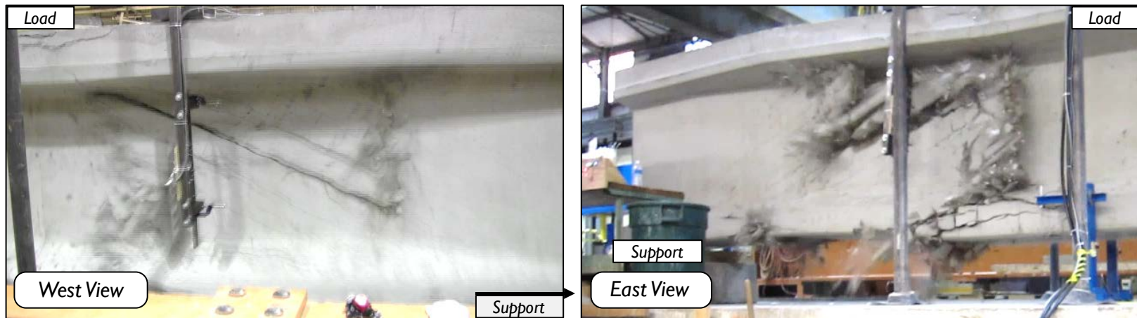
(B) Control Specimen (Tx62-3(S)): Immediately After Shear-Compression Failure
