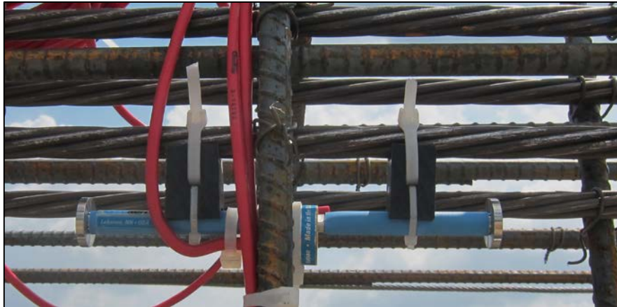
Figure 3-26: Vibrating Wire Gauge Attached to Top Strands
