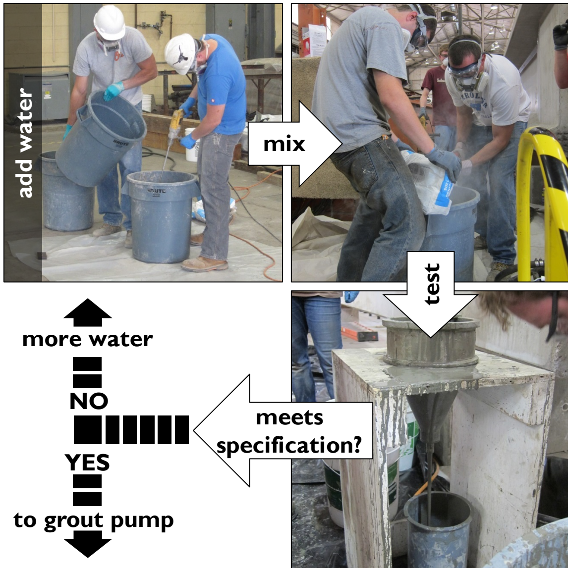
Figure 3-23: Grout mixing procedure
