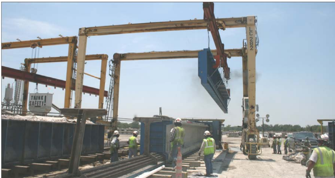
Figure 3-18: Removal of Side Forms Prior to Prestress Transfer
