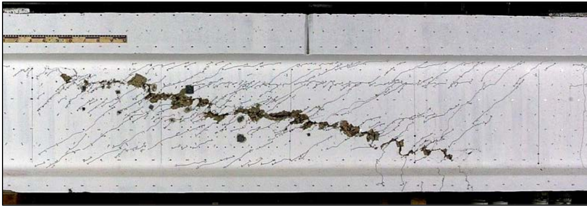
Figure 2-18: Local Crushing Along the Trajectory of the Duct (Ruiz & Muttoni, 2008)
