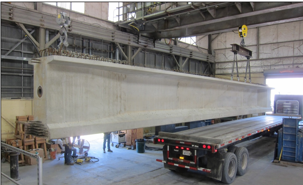
Figure 3-20: Two Crane Lift System at FSEL
