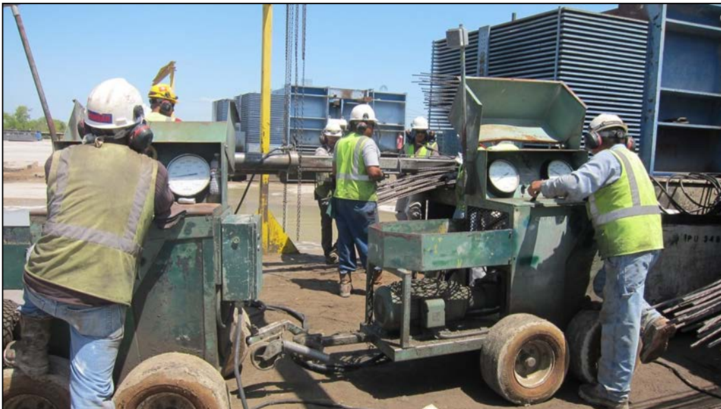
Figure 3-14: Individual Stressing of the Pretensioning Strands at Fabrication Plant
