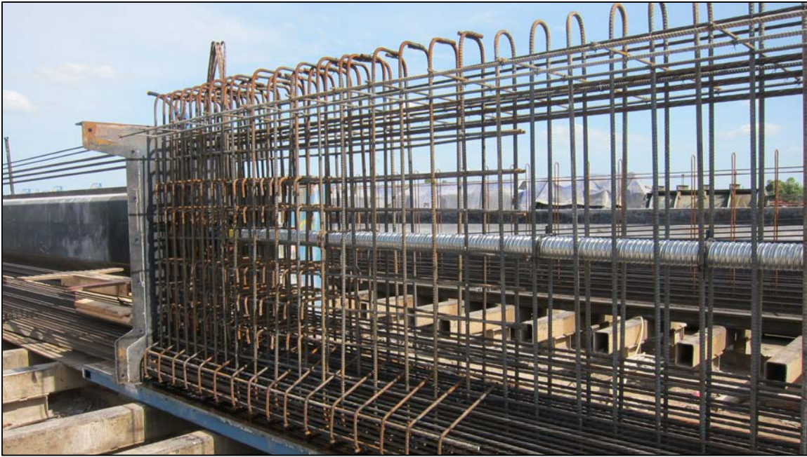
Figure 3-16: End-block reinforcing cage of Tx62-7
