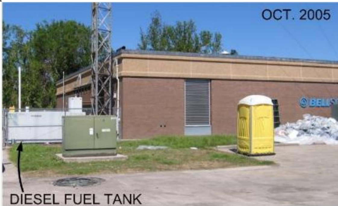
Fig. 7.1. Central office during Katrina with diesel fuel tank
