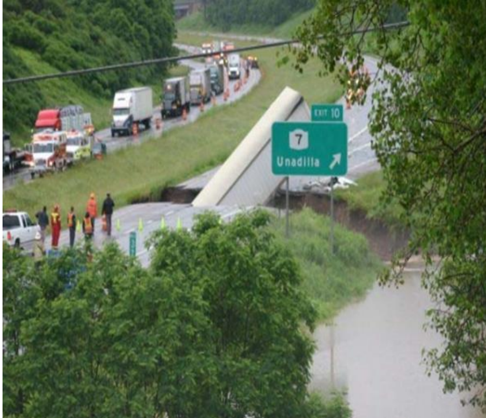
Figure 2.1 Culvert failure on Interstate-88 in New York (New York State Police Department, June, 2006)
