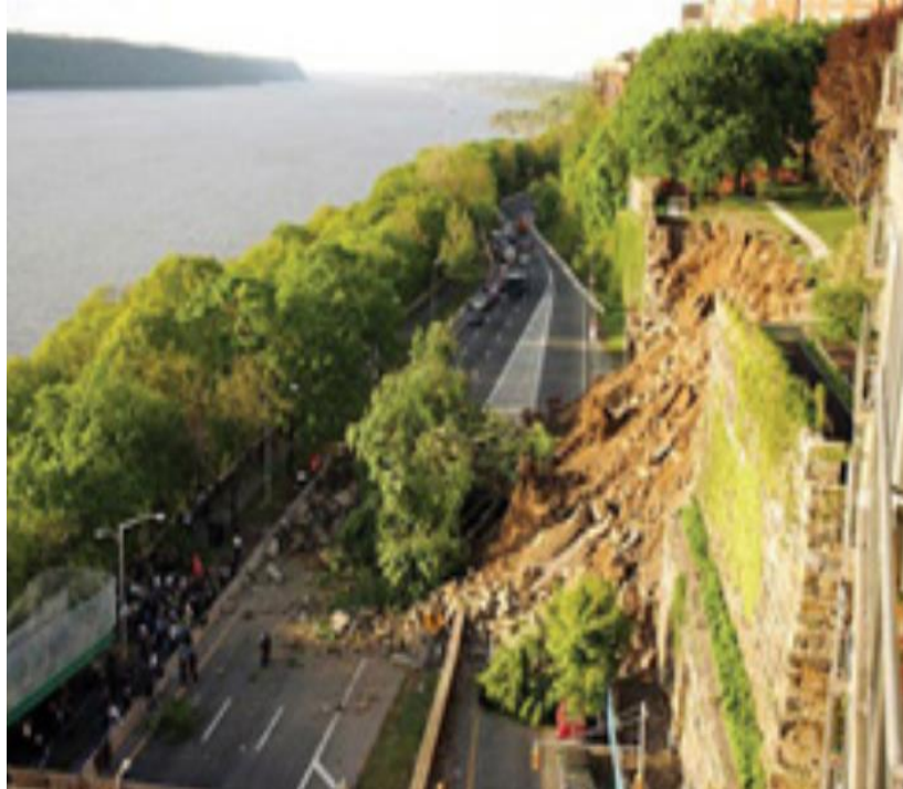
Figure 2.2 Failed ERS along Riverside Drive near Manhattan in New York (The New York Times, May 13, 2005)
