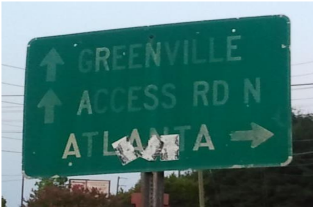
Figure 2.5 Example of a Failing Road Sign
