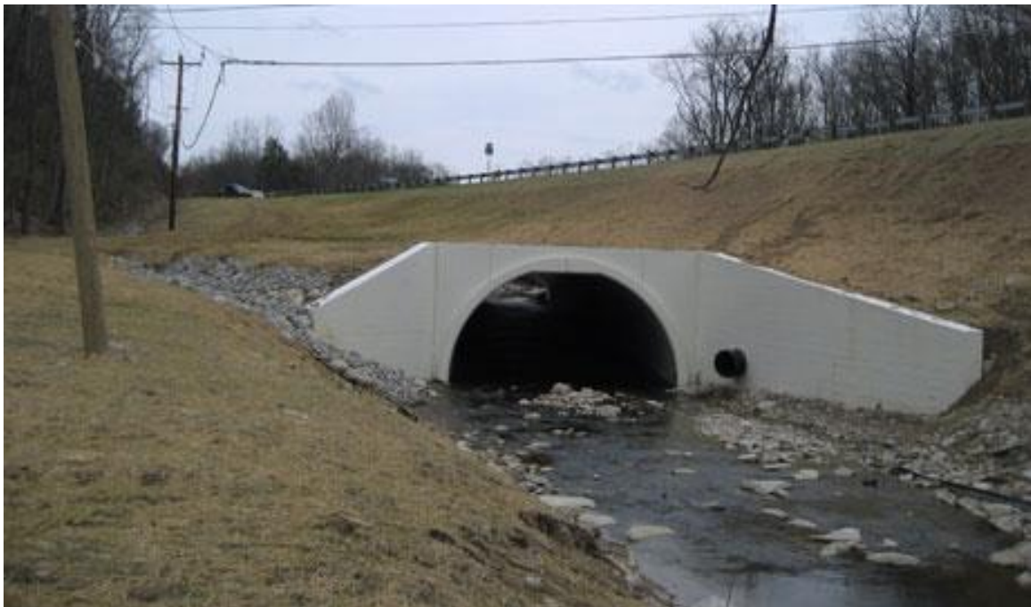
Figure A.2 Example of a Cylindrical Culvert
