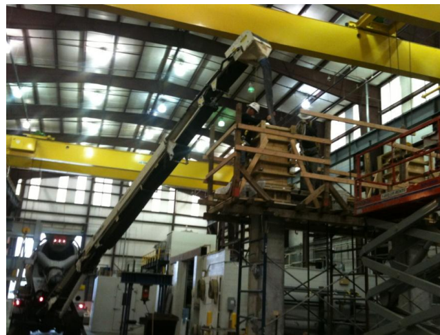
Figure 101: Conveyor used to pour the top half columns
