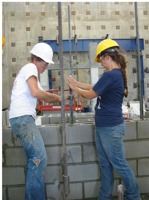
Figure 117: Splicing vertical reinforcement
