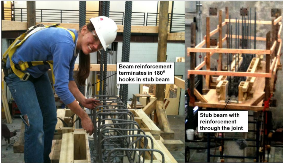
Figure 100: Construction of the beams
