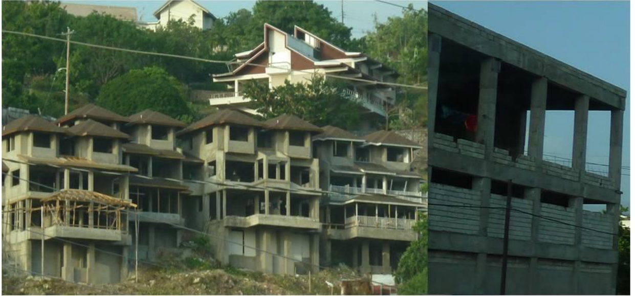
Figure 4: Condominiums (left) and close up of CMU infill wall (right) under construction in Jamaica
