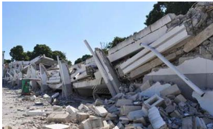
Figure 2: Soft story collapse observed during the 2010 Haiti Earthquake (DesRoches et. al. 2011)
