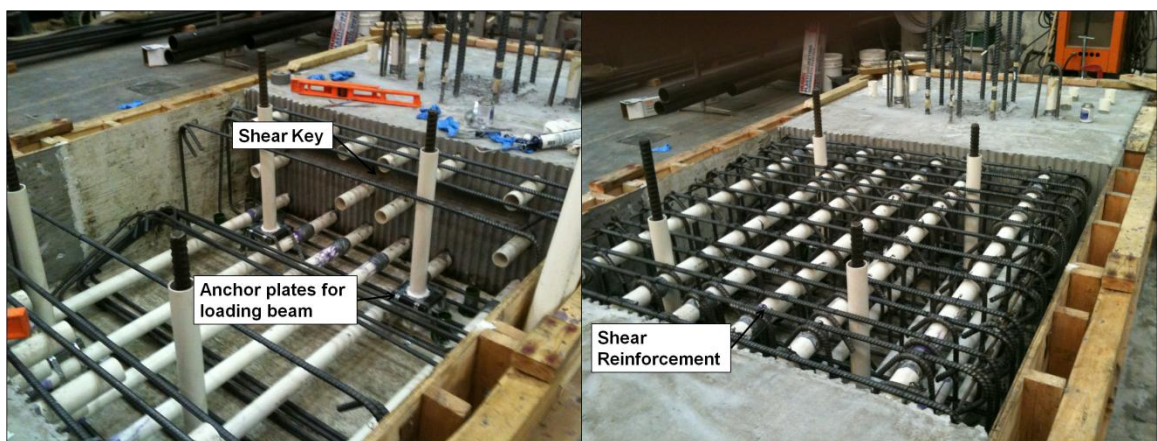
Figure 96: Construction of the post-tensioned slab, continuing with the middle section
