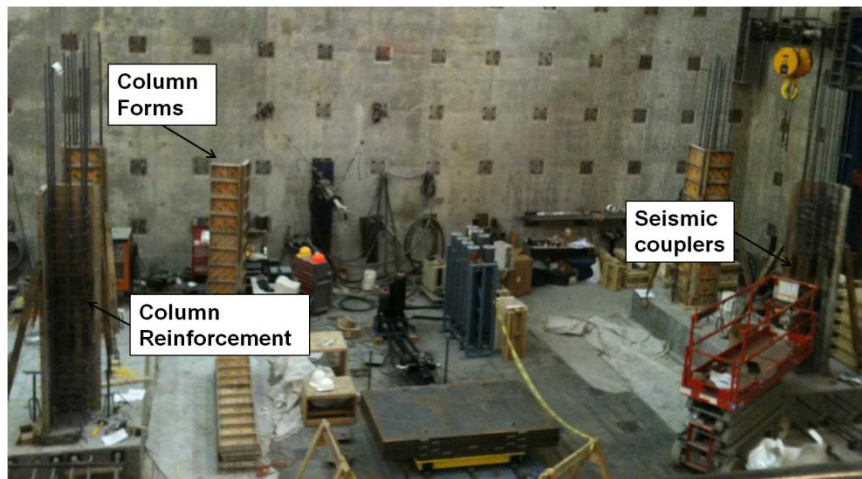
Figure 97: Installation of column forms and reinforcement
