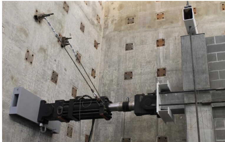
Figure 123: Hydraulic used to apply lateral loads and stiffened plate on left side of loading cage
