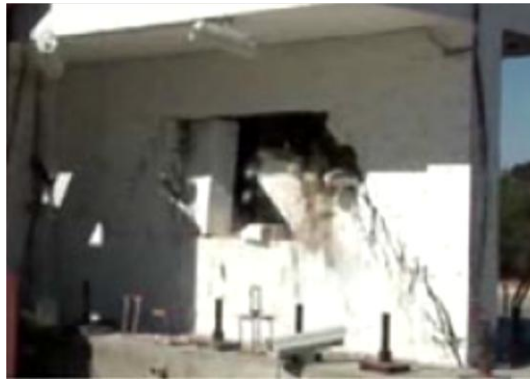
Figure 18: Large diagonal crack formed during shake table test (Stavridis et. al. 2012)
