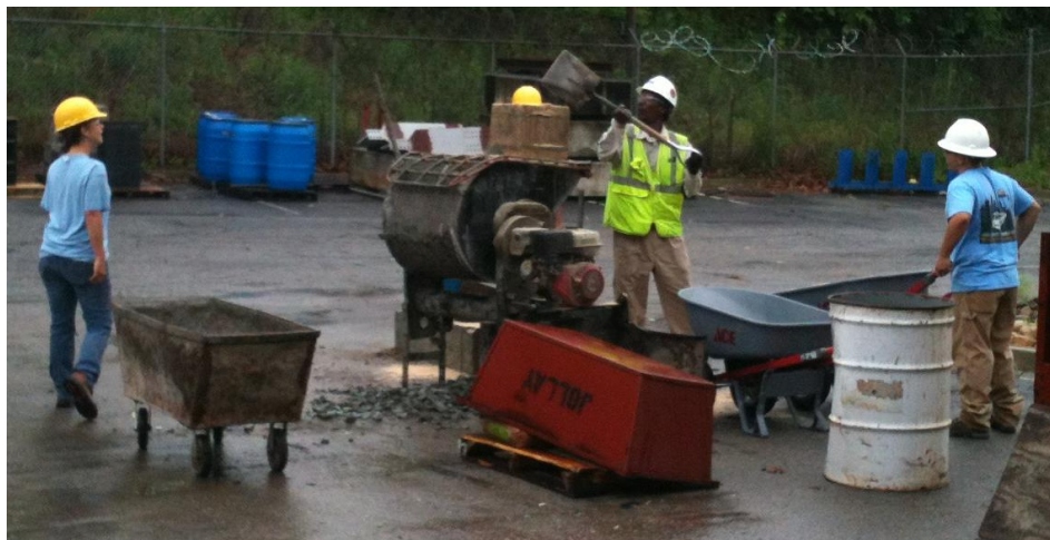
Figure 112: Volumetric batching of the mortar
