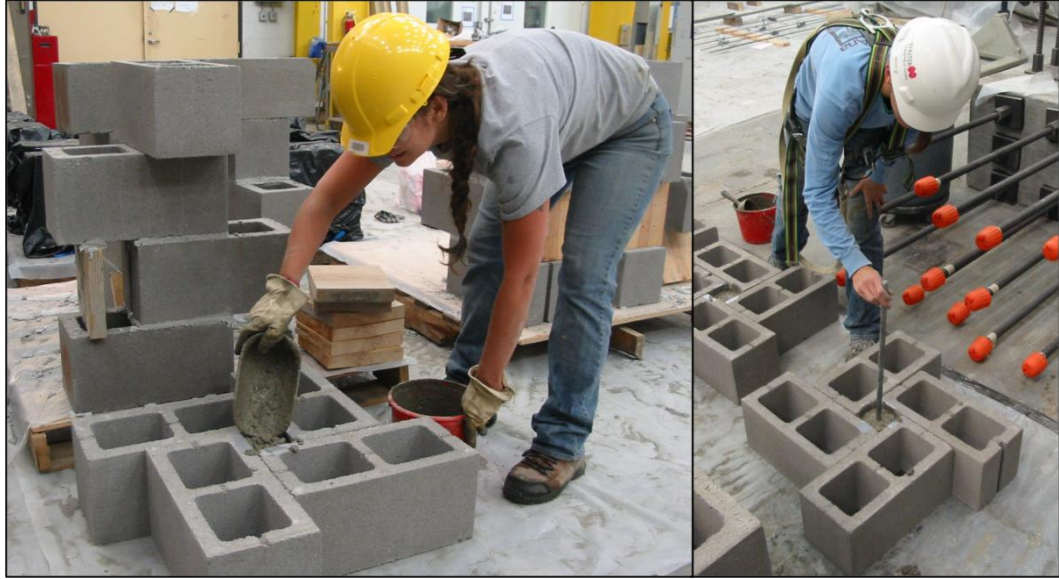
Figure 108: Construction of grout prisms made from weak concrete
