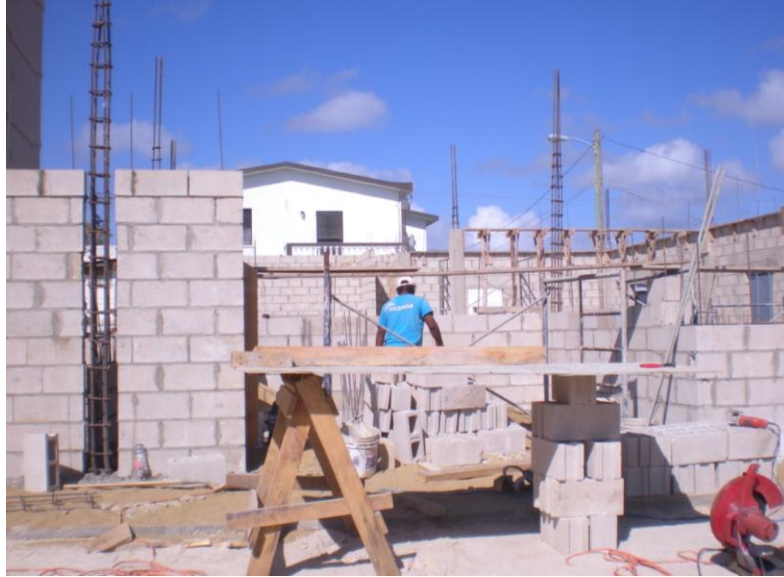
Figure 6: Typical Belizian construction, placing column rebar and the infill wall
