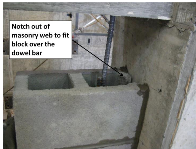
Figure 118: Dowel reinforcement extending down from the RC beam
