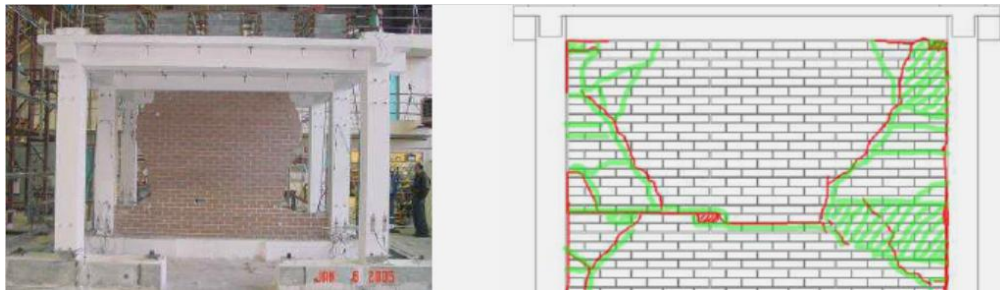
Figure 16: Unreinforced masonry wall test showing interface cracking and bed joint sliding (Mosalam 2005)
