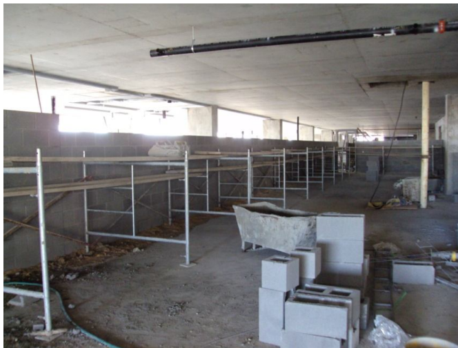
Figure 22- Scaffold to build a long straight wall
