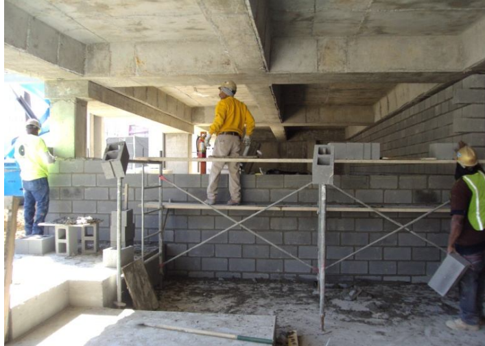
Figure 19- Long straight block wall with two masons (left) and one laborer
