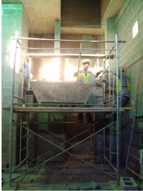
Figure 20- Mason and laborer working on a short block wall
