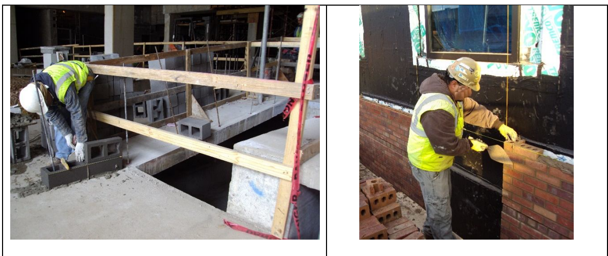
Figure 8a- Mason laying block; Figure 8b- Mason laying brick
