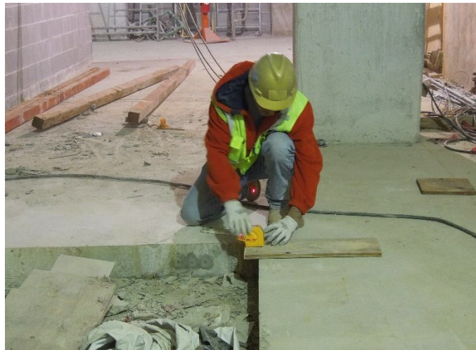
Figure 13- Foreman using the laser to lay out a wall
