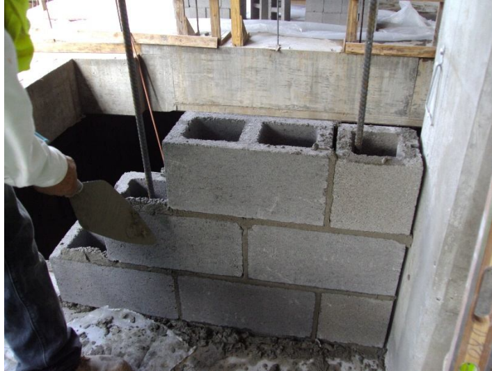
Figure 34 –Mason building the lead in a block wall
