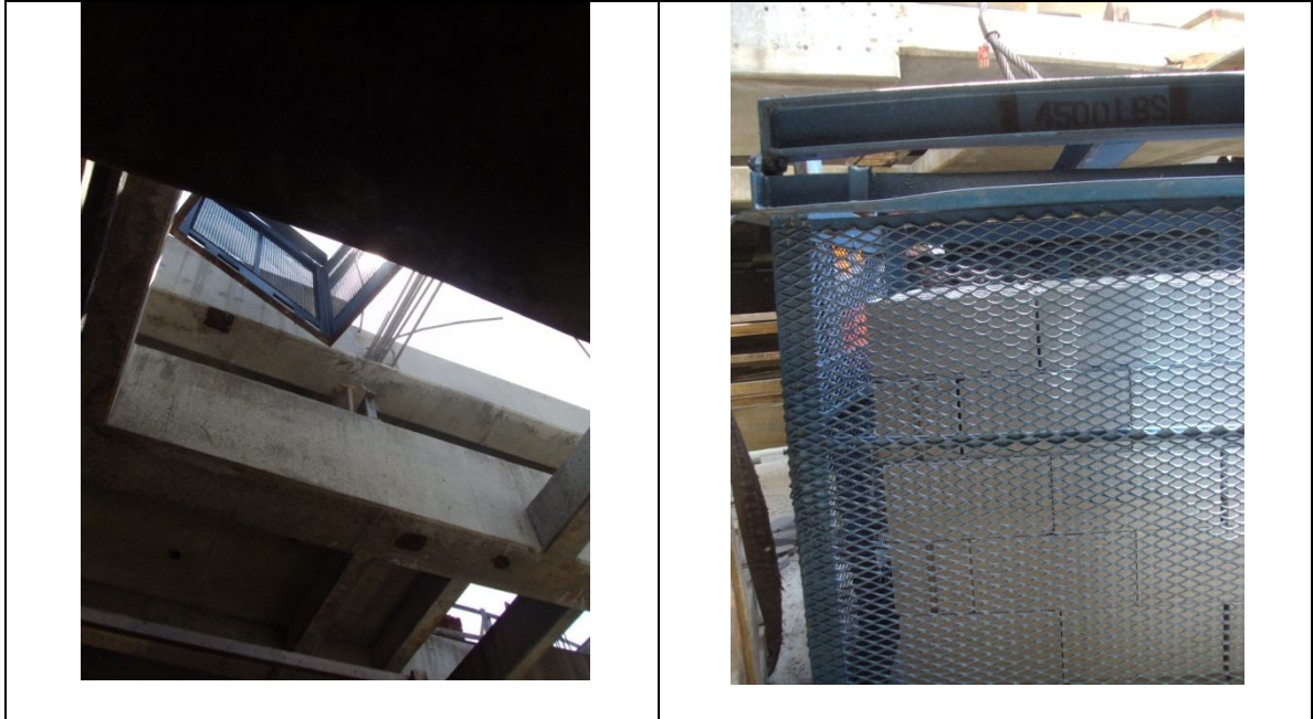
Figure 18a, 18b- Crane used to lift a metallic cage with blocks
