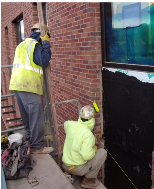
Figure 33- Masons putting the pole line in a brick veneer wall
