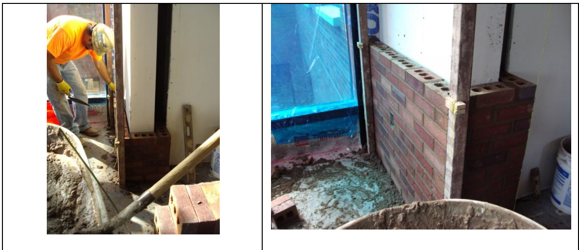
Figure 10- Mason working in an interior column.
