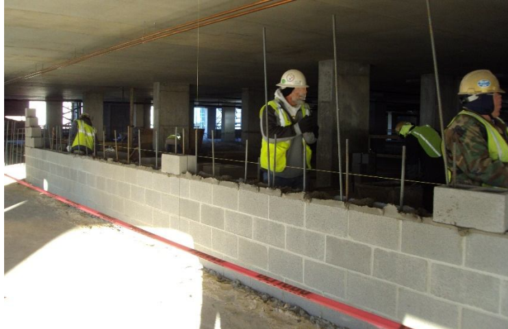
Figure 15- Three masons and two laborers working on a block wall
