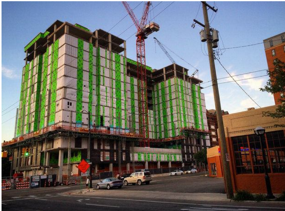
Figure 45- North façade of the building
