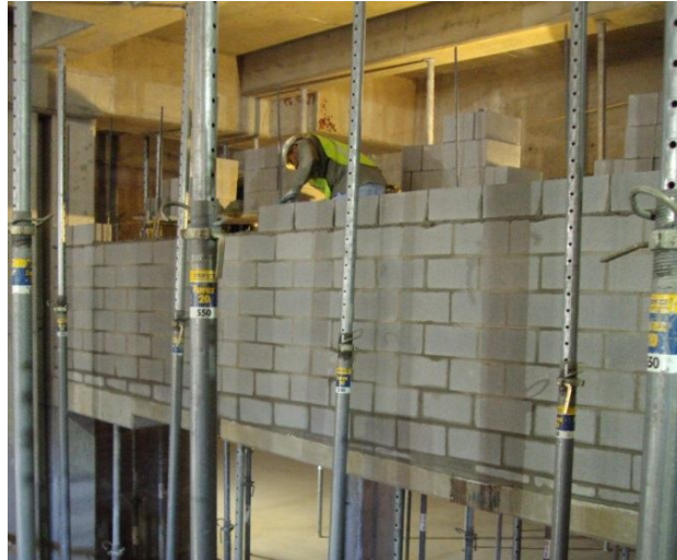
Figure 31- Mason working on a long straight block wall
