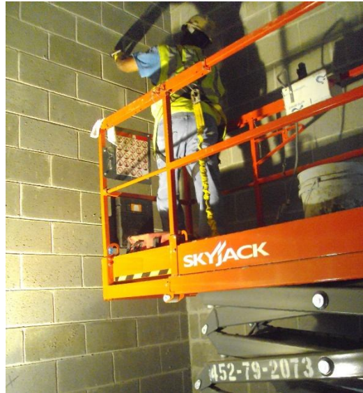
Figure 16- Mason cleaning the surface of the blocks and finishing joints
