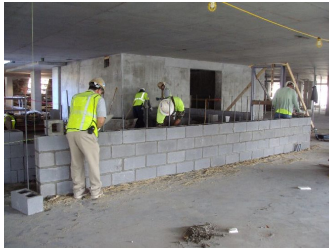
Figure 26- Four masons (and laborer) on an L-shaped block wall
