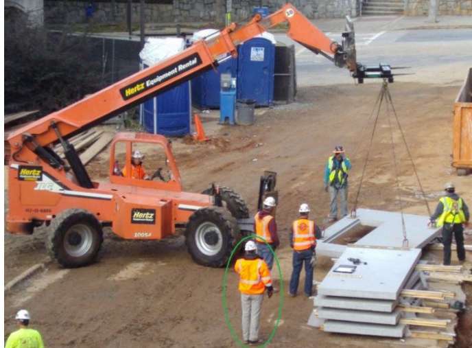
Figure 4- Superintendent on the site overseeing the installation of stone pieces
