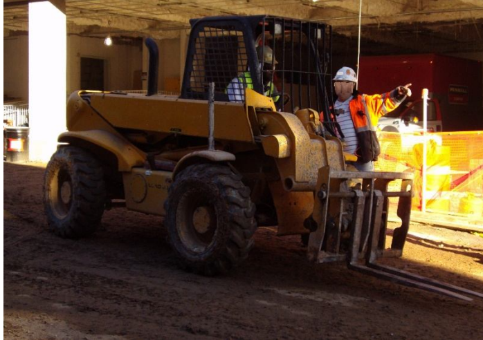
Figure 5- Foreman (right) giving instructions to the forklift operator
