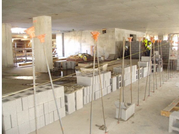
Figure 14- Wall ready for the masons
