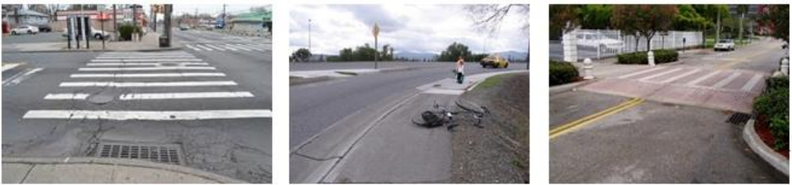
Figure D12 Examples of Crosswalk (Left: Marked, Center: Unmarked, Right: Raised)
