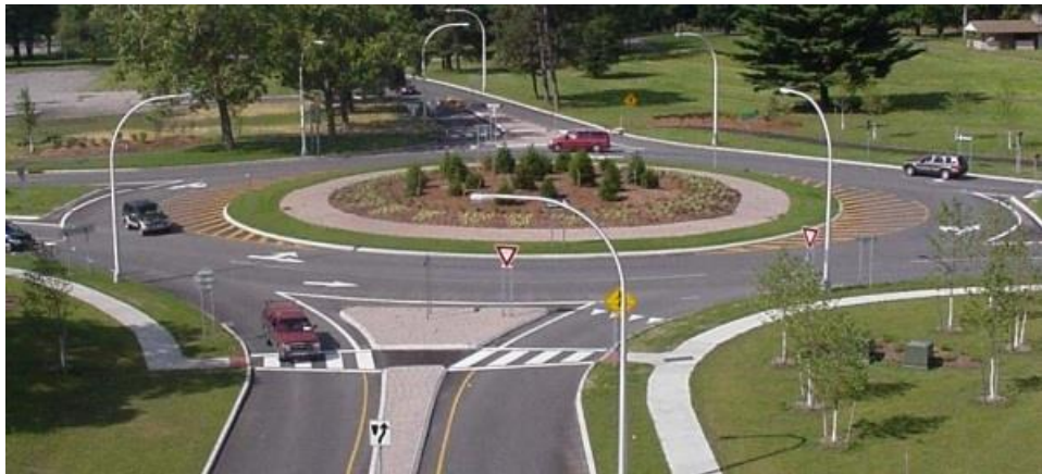
Figure 10 Raised Splitter Island with Flared Ends and a Raised Central Island at Roundabouts
