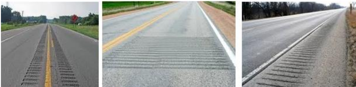
Figure D15 Examples of Rumble Strips (Left: Centerline Rumble Strips, Middle: Lane Rumble Strips, Right: Shoulder Rumble Strips)
