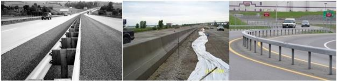
Figure D9 Examples of Median Barrier
