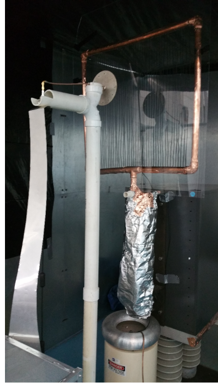
(b) Stand with antenna at HV test set
