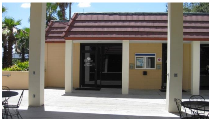
Figure 3.12. Newly renovated music building in 2013. Photograph by author.
