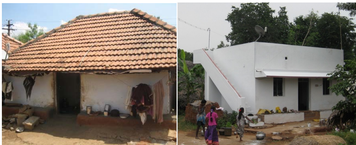
Figure 17. Examples of typical house with tile roof (top) and cement roof (bottom)
