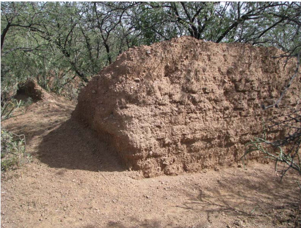
Figure 12.32. Melted historic, adobe-brick, structure at Los Argüelles.
