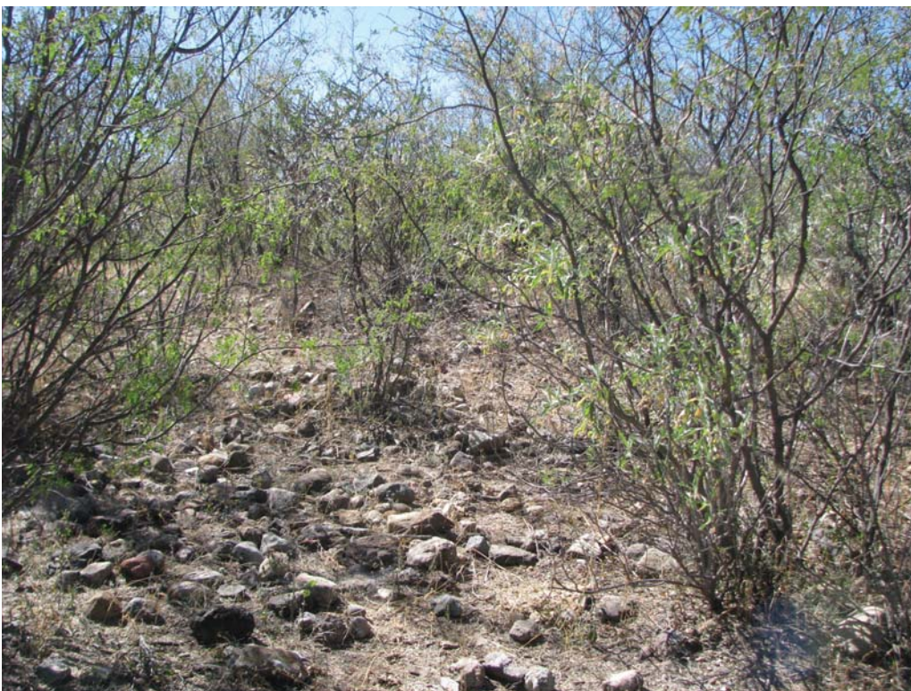
Figure 12.2. A deteriorated structure likely of adobe and river cobbles at Las Clavellinas.
