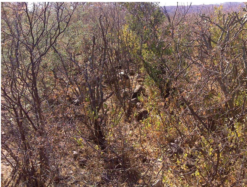
Figure 12.3. The large wall foundation at Las Clavellinas on the edge of the mesa (mostly obscured by vegetation).
