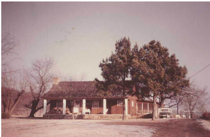
Figure 10. Farm in Mansfield Arkansas.
