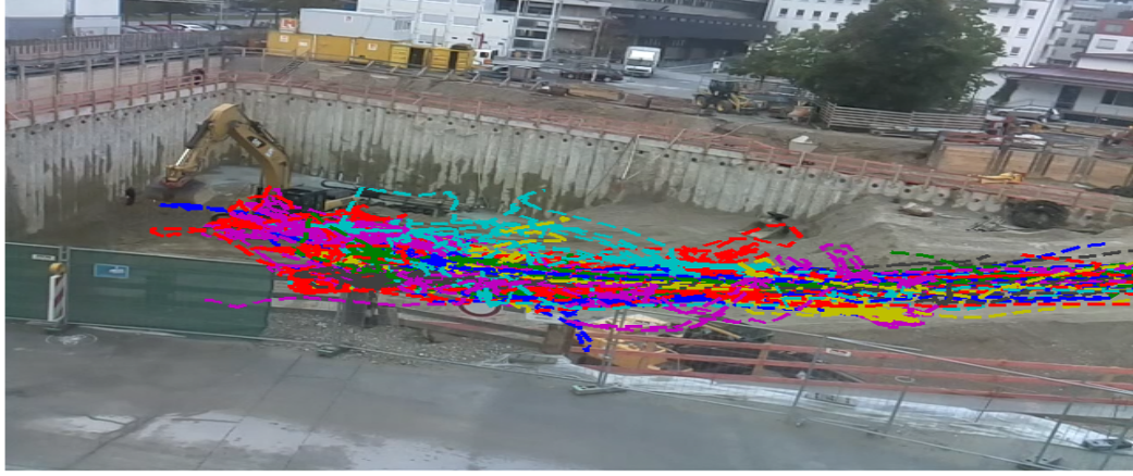
Figure 41: Tracking results for day 11 of the translaTUM construction site.
