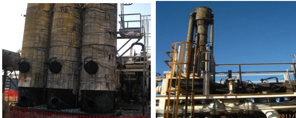
Figure 4.8 – Fire Rebuild Gas Plant - Oklahoma (Rainbolt 2014)
