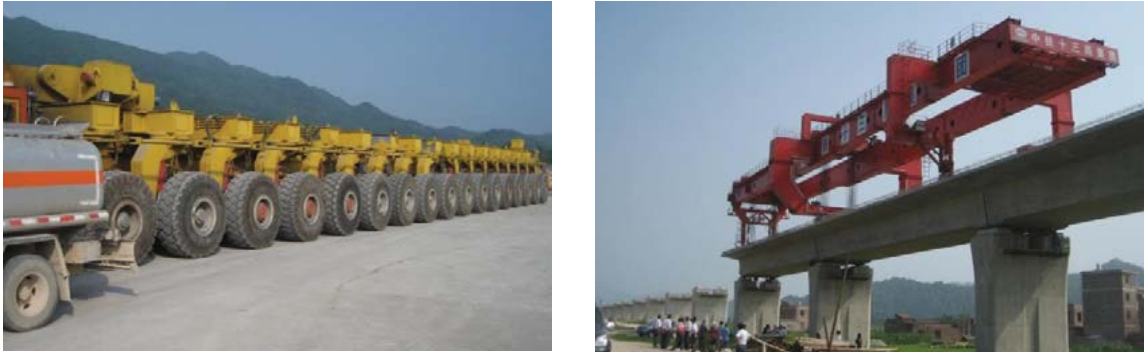
Figure 4.10 – Chinese High Speed Rail, Beam Carrier and Launching Equipment (Ollivier 2014)
