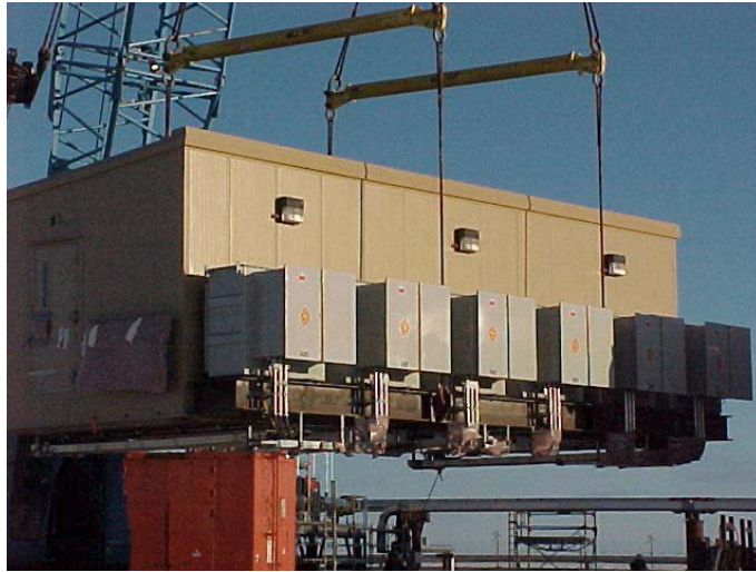
Figure 4.7 - West Sak, Pump Drive Module Setting (Garrett 2014)
