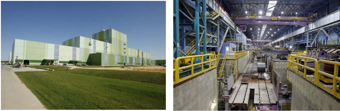
Figure 4.3 - ThyssenKrupp Hot Dip Galvanizing Line, near Mobile Alabama (Mitchell 2012, Finch 2014)
