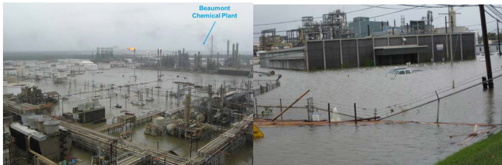
Figure 4.9 - ExxonMobil Chemical Plant, Hurricane Ike Recovery Effort (Critzler 2015)
