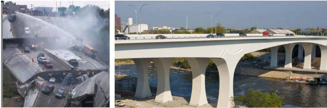
Figure 4.1 - Saint Anthony Falls, I-35 (Lestrud 2112, R.J Watson 2015)
