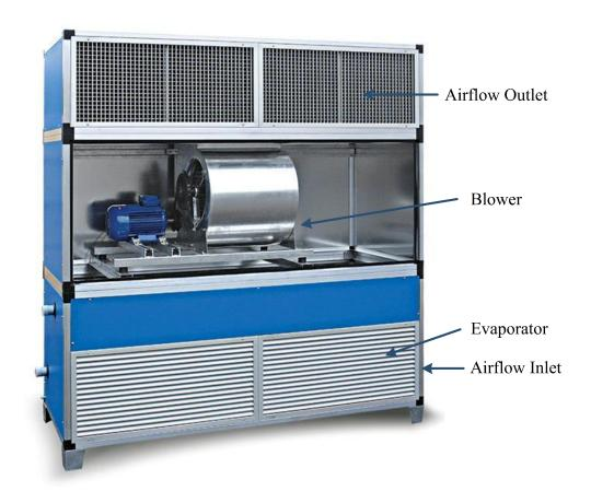
Figure 6.10 The experimental AHU in this dissertation.
