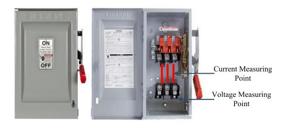
Figure 6.13 Measuring points at disconnected box.
