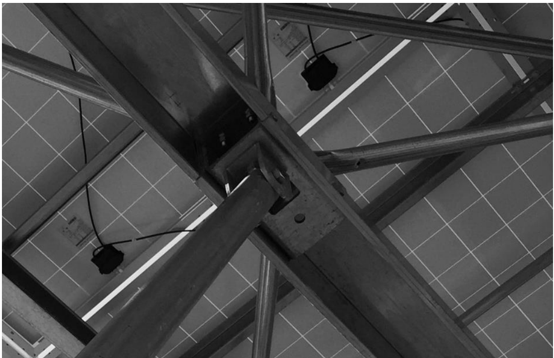
Figure 116: Studied QuadPod assembly after fabrication and erection
