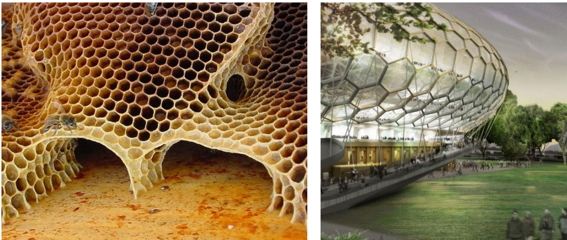
Figure 3.1: Left: Natural honeycomb. Right: Design by E. van Egeraat based on a hexagonal torsion-free support structure.
