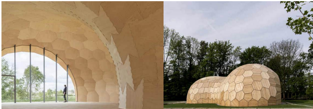
Figure 4.2: A planar-hexagonal pavilion constructed with wooden panels [34].
