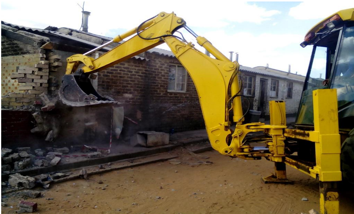
Figure 3.1: Dilapidated hostel building in Diepkloof
