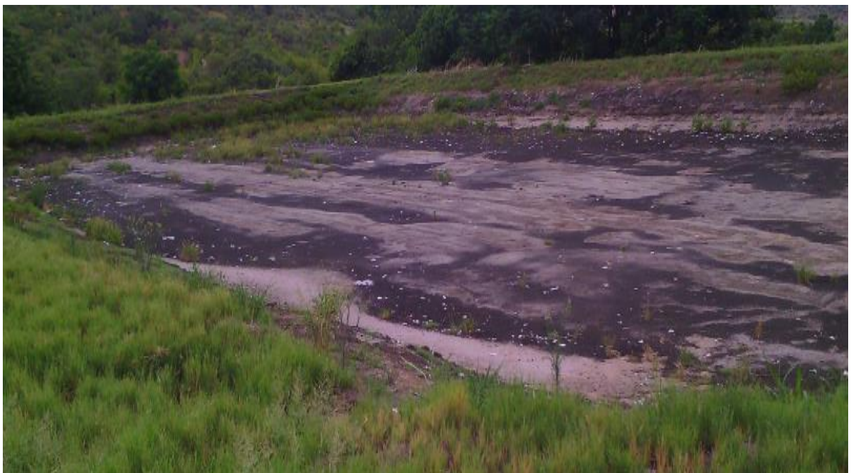
Dried up stabilization pond
