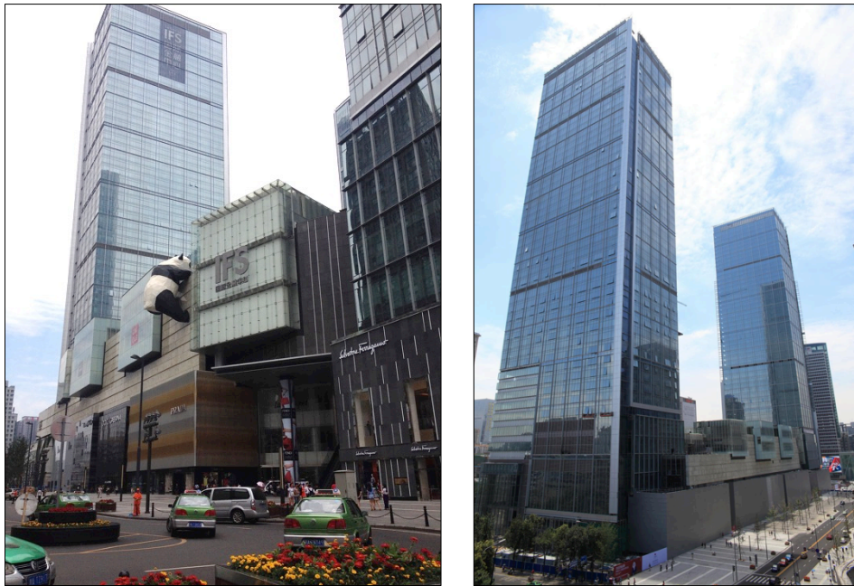
Figure 4.8 The International Finance Square in Chengdu. Source: Photos taken by the author.
