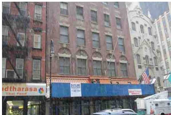
Fig. 8: Washington Street with the former St. George’s Church.
