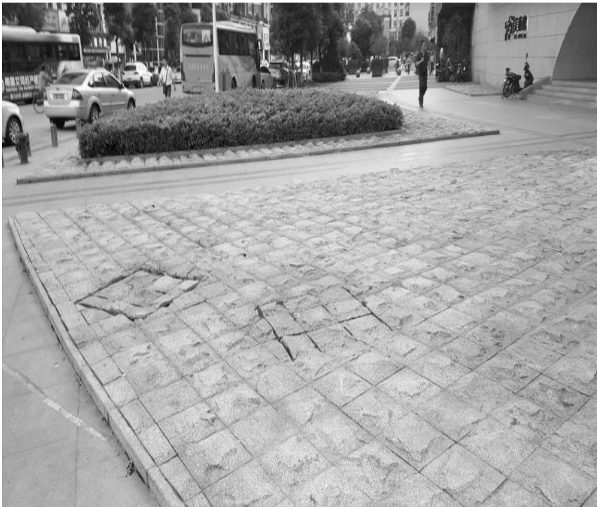
Figure 27. Anti-street vending architecture along Wuwei Street. Source: Author.
