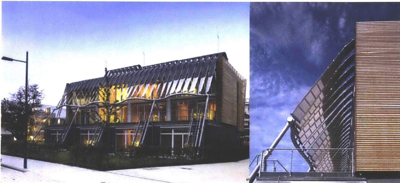
Figure 4.32. Soft House with responsive solar textile screen, International Building Exhibition, Hamburg, Germany (2013). http://a2.images.architettura-italiana.com/image/upload/c_fit,w_1440/f_auto,q_80/v1/project_images/4000971/SoftHouse_102.jpg .
