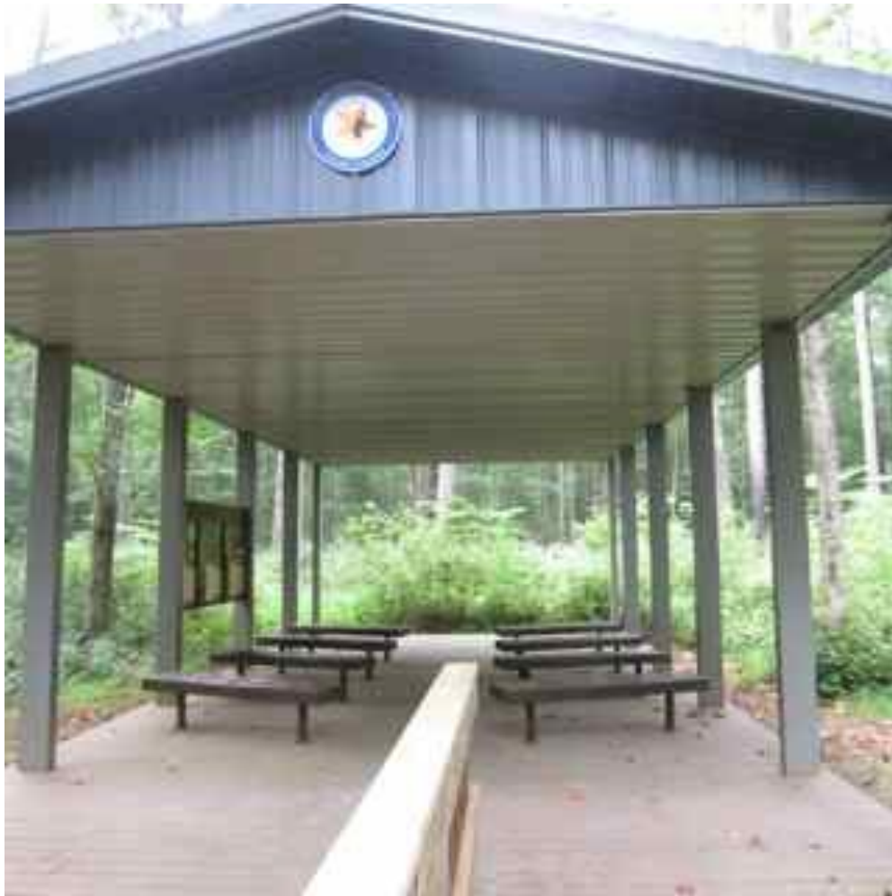
Figure 11: Photo of the Underground Railroad Pavilion.
