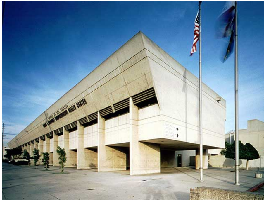
Figure 5.3 Top: Architectural rendering of Hubert Humphrey Comprehensive Health Center, originally known as the Southeast Comprehensive Health Center, or the “Slauson and Main” clinic (after the major cross streets located nearby). Below: Completed Center, photo date unknown.
