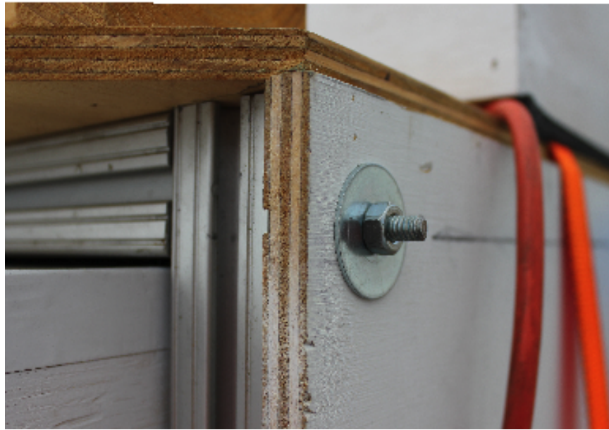
Figure E.8: Threaded rod for connecting the enclosure panel to the 8020 frame.
