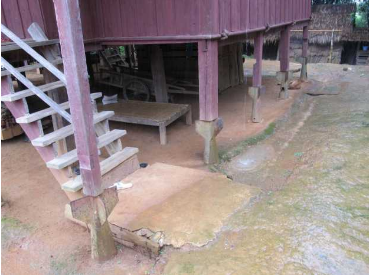
Figure 2.3 Dismantled general purpose bombs used as supports for a stilt house near Phonesavanh, Xieng Khouang Province. Source: Author.
