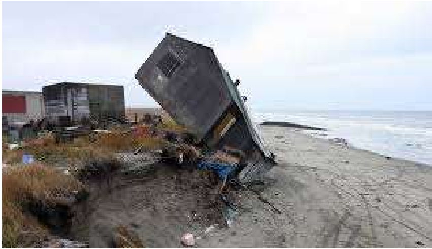
Figure 1.1 Shishmaref: Abandoned house sits on the beach after sliding off during the 2005 fall storm. Credit: Diana Haecker/AP
