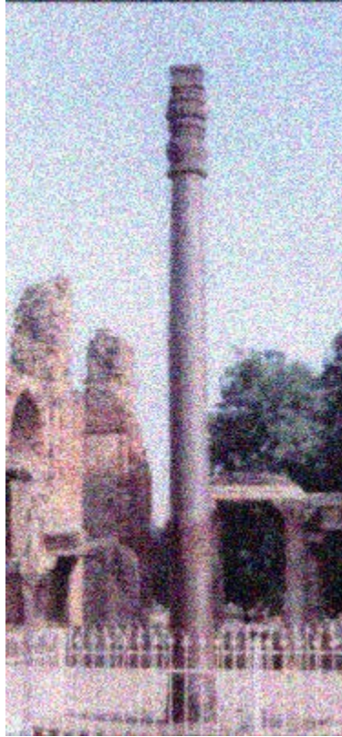
Figure 1.1: The Iron Pillar of Delhi. The chemical composition of this iron pillar, specifically its P-content (0.15 at. %), has rendered its resistance to corrosion for approximately sixteen centuries. The excellent corrosion resistance has spurred interest in the corrosion behavior of various iron-alloys.
