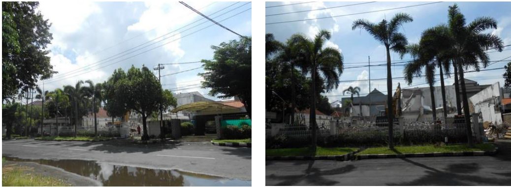
Figure 4.4 One of the listed buildings has been completely demolished; this is clearly against the law Source: Author's fieldwork, 2014
